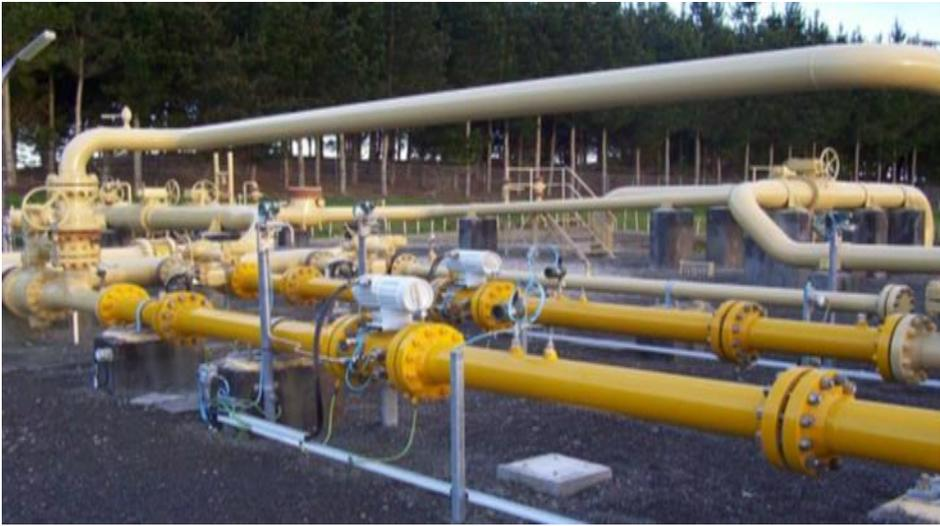
**Figure 5 - two ultrasonic meter streams**
