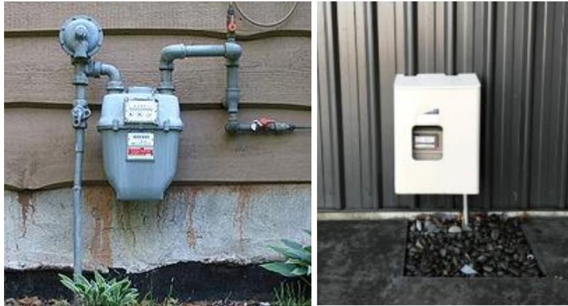
**Figure 7 - Residential gas meter installation**
